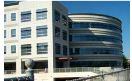
Existing Arlington building.
