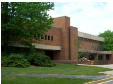
Additions to the University's Aquatic Center and Physical Education building are planned to support enrollment growth.
